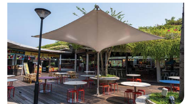
■ One of the new solar canopies at Satay by the Bay
